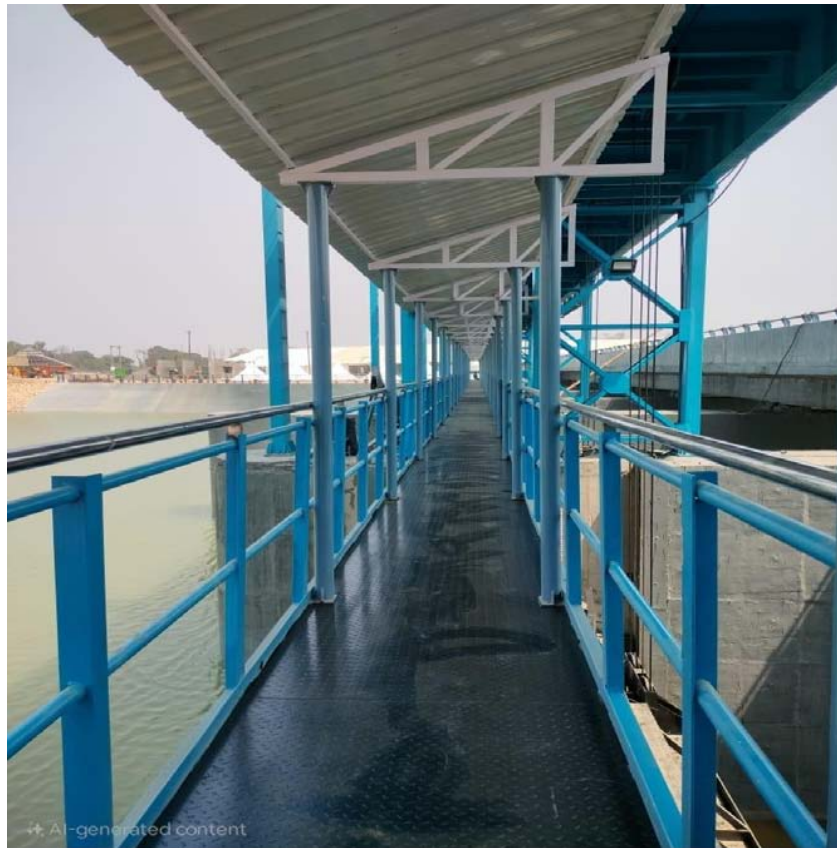
Figure 3: Upstream Inspection Pathway
