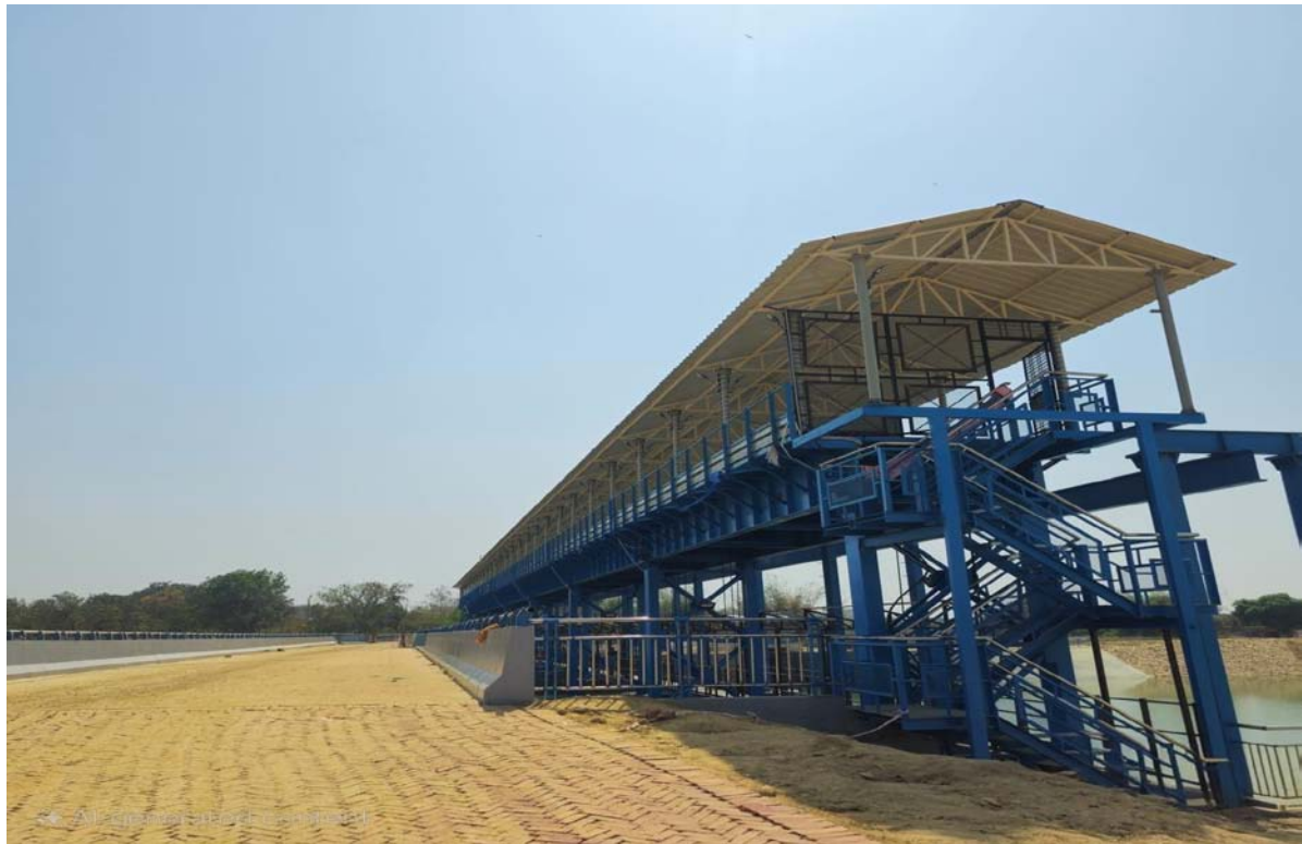
Figure 1: Photograph of the Rohin Barrage
